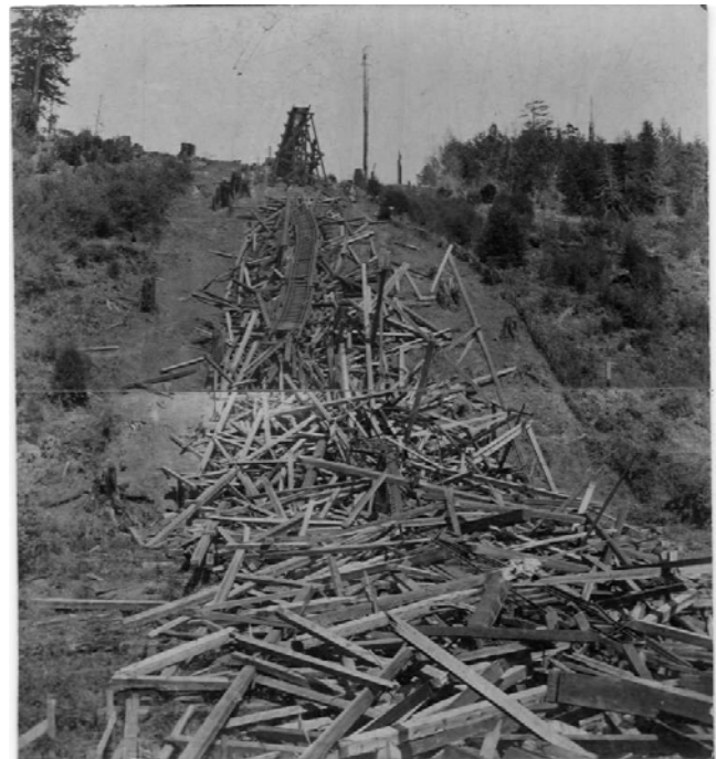
Eastern Railroad's 146 foot high, 1000 foot long trestle over Jughandle Gulch on morning of 1906 earthquake. It was immediately rebuilt. FB-MCHS, MCM
